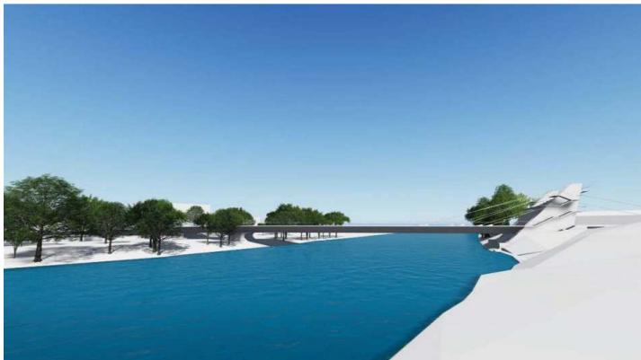
The concept of a new bridge to the core of the site sets a minimalist silhouette. It is visually connected by high-growth massifs that, on the right bank, obscure a carrier pylon with a vantage point. The aforementioned structural element is placed on the right side of the river bank, so that this vertically expressed element is further away from the protected area of Kastel fortress and the river ambient next to Kastel fortress.
