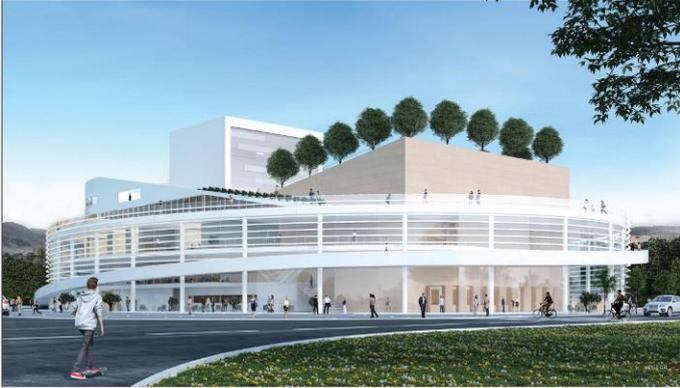
The structure is a centrally organized spatial-form structure with a core formed from the basic purposes of the building and a circular hall that surrounds the core. The roof plane is treated as an additional space of contents complementary to those required by the tender. A special quality of the proposed solution is the direct connection of the ground with the roof with a pedestrian ramp, which, in addition to the communication role, also becomes a kind of a viewpoint.
