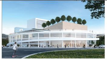
The structure is a centrically organized spatialform structure with a core formed from the basic purposes of the building and a circular hall that surrounds the core. The roof plane is treated as an additional space of contents complementary to those required by the tender. A special quality of the proposed solution is the direct connection of the ground with the roof with a pedestrian ramp, which, in addition to the communication role, also becomes a kind of a viewpoint.
